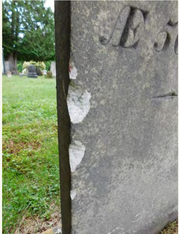
Figure 3. Gouges from lawnmower strikes on a marble stone from Cortland County.
