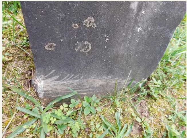
Figure 7. An example of weed eater damage on a marble stone from Cortland County.
