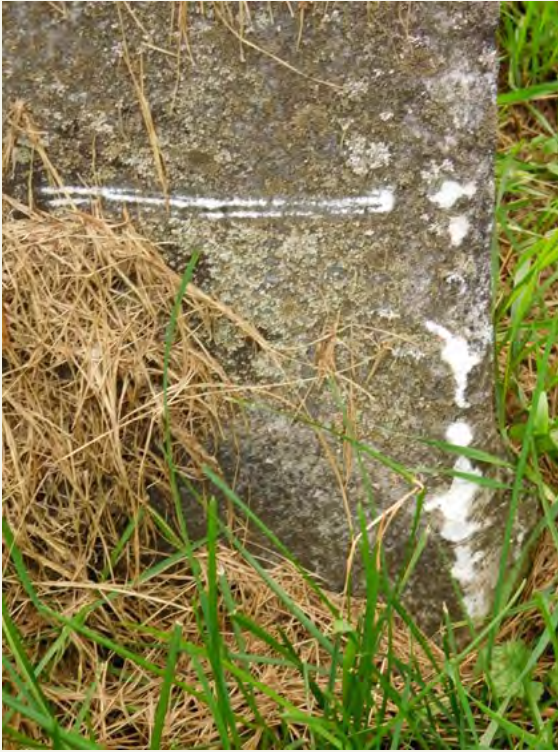
Figure 5. Lawnmower scrapes and gouges on a marble stone from Cortland County.
