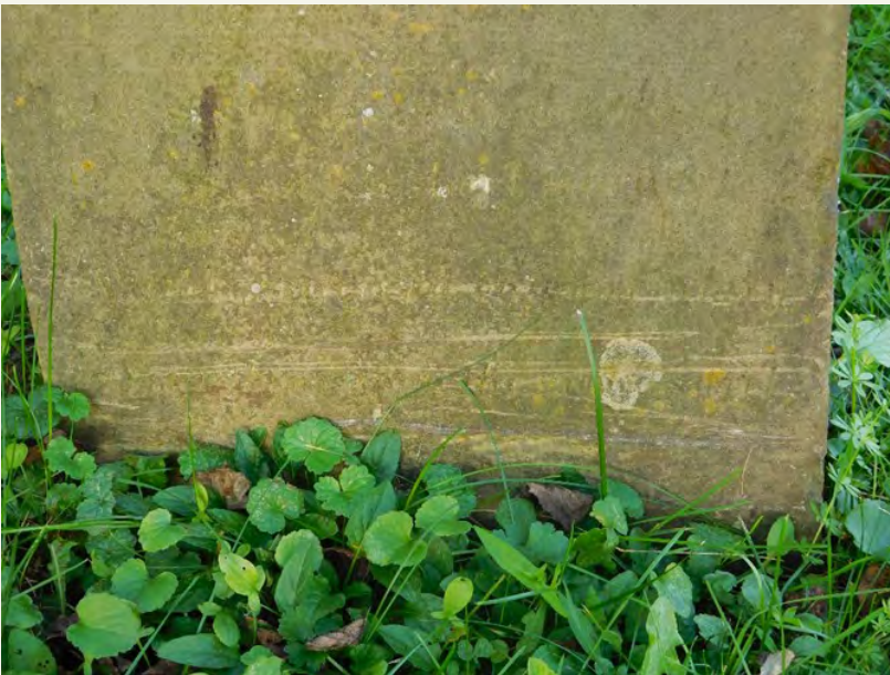
Figure 4. Lawnmower strikes on a sandstone marker from Cortland County.
